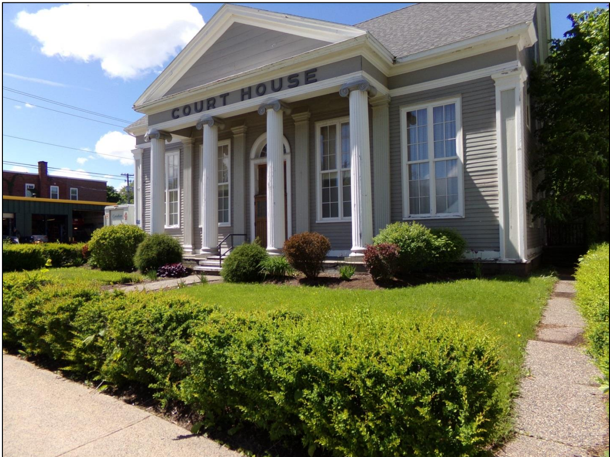
Figure 1: Photograph of the Antigonish County Court House, taken 2016
